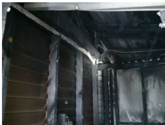
'Free' roof truss
