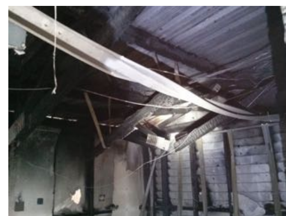
'Fixed' roof truss
