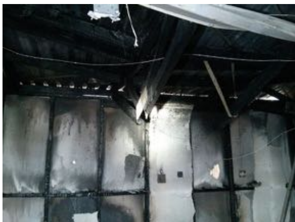
'Centre' roof truss
