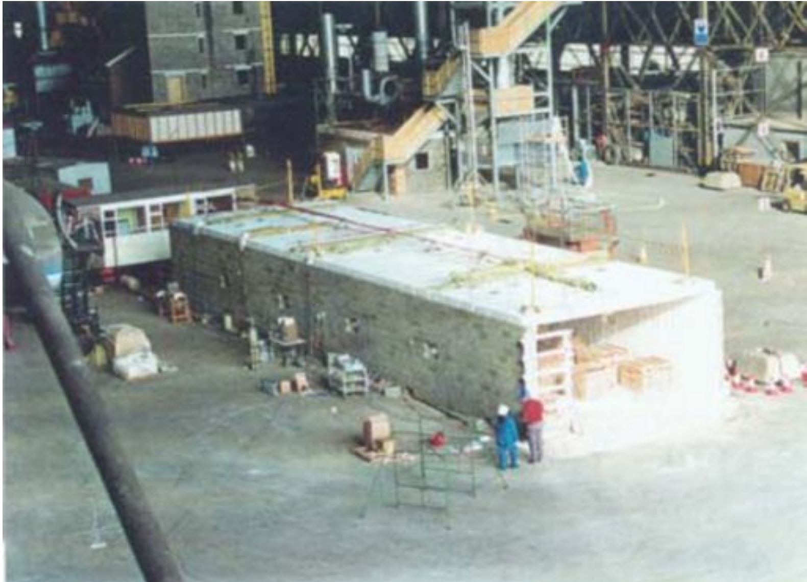
The 23 m long fire compartment at Cardington around 1993
