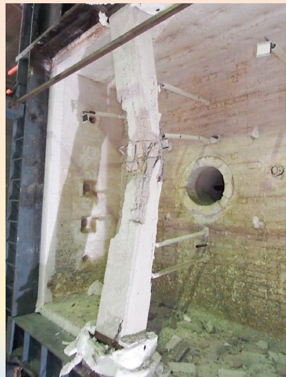
Thomas Gernay, Jean-Marc Franssen, Fabienne Robert, Robert McNamee, Roberto Felicetti, Patrick Bamonte, Sven Brunkhorst, Siyimane Mohaine, Jochen Zehfuß, Experimental investigation of structural failure during the cooling phase of a fire: Concrete columns, Fire Safety Journal , Volume 134, 2022,
