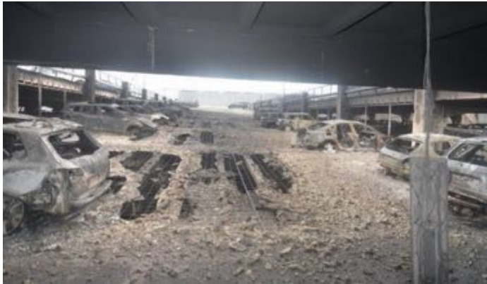
Fire in Multi-Storey Car Parks - Feb 2018
