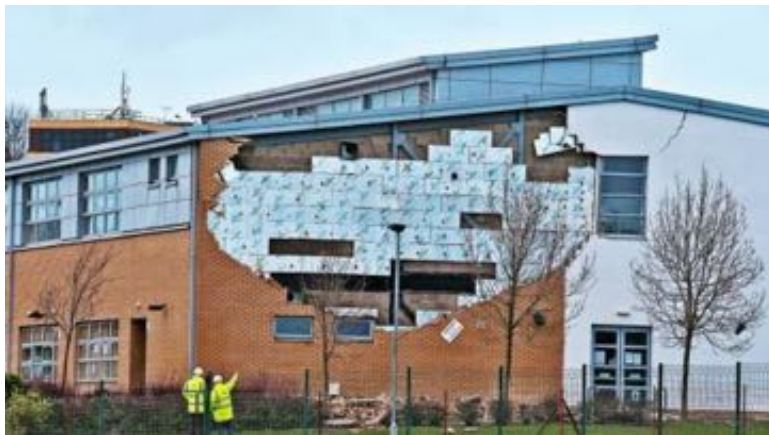
Construction of Edinburgh Schools - Feb 2017
