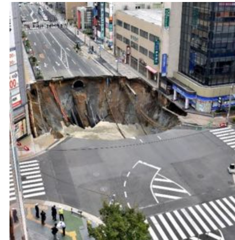
Sudden loss of ground support - July 2017
