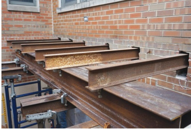
The Journal of Light Construction – Opening Up a Masonry Wall
