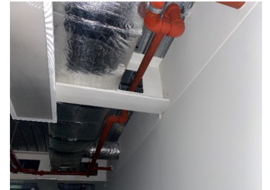
Steel beams protected with thin intumescent paint
