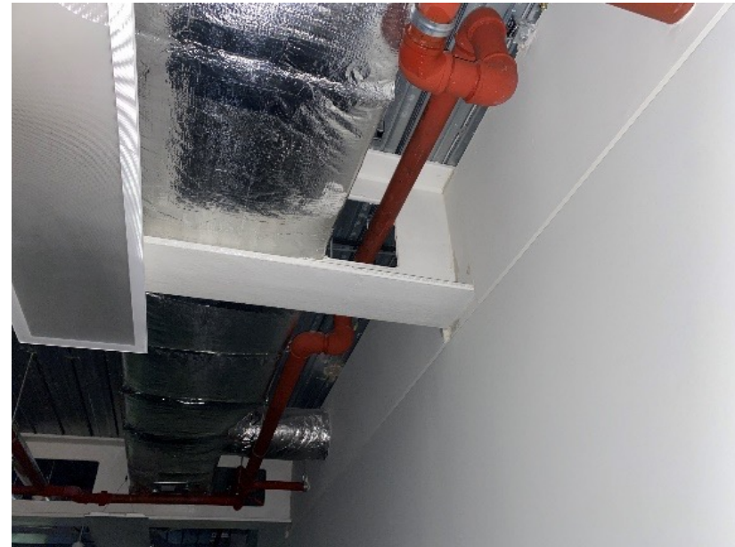
Steel Beam protected with intumescent coating
