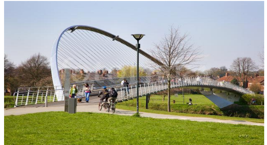
Millennium footbridge, York, UK. Welded duplex sections. (SCI, 2017)
