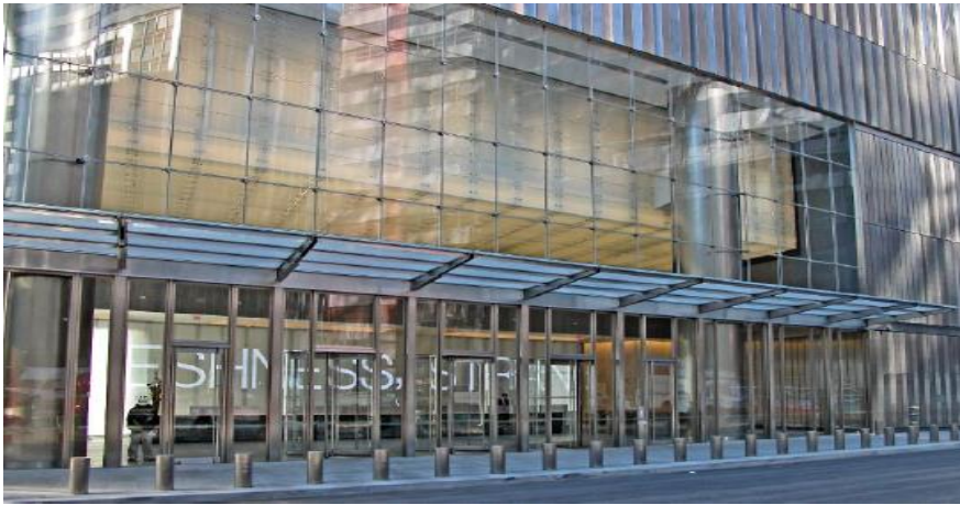
Stainless steel columns, entrance canopy at Seven World Trade Centre, New York (SCI, 2017)
