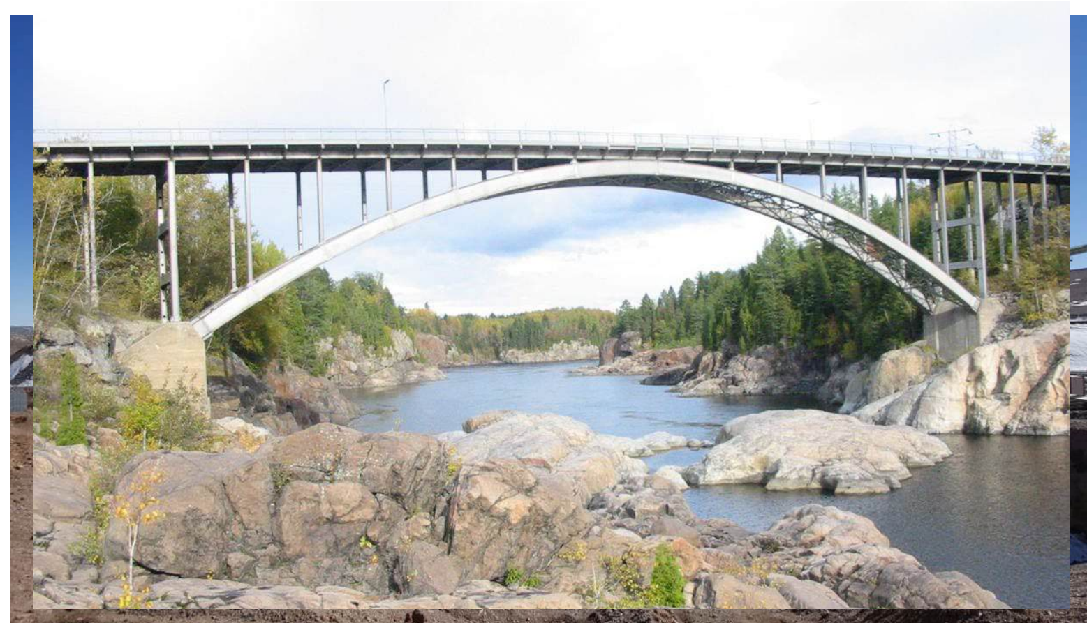
Arvida bridge, Quebec, Canada [5]
