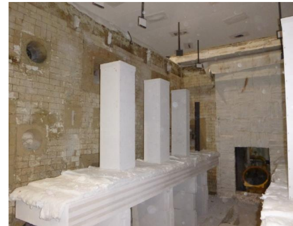
Short columns after cooling down (protection intact)
